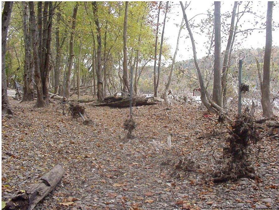
Photograph 6: Fence with flood debris on the western portion of the Crown Vantage Landfill site, August 11, 2005
